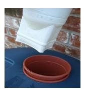
Let all glue dry before exposing it to water. Be sure that the site for the rain barrel is flat, or level it with sturdy materials such as bricks or cinder blocks. Water weighs roughly 8 pounds per gallon, so you won't be able to move the barrel when it is full, and on sloping ground it might tip.
