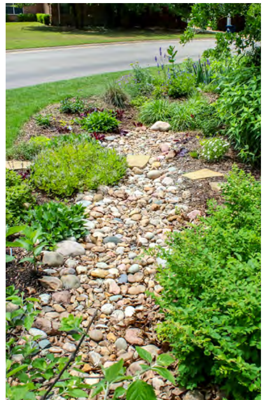
This Dry Riverbed, built to address control of excess runoff, provides a pathway for rainwater into the raingarden.
